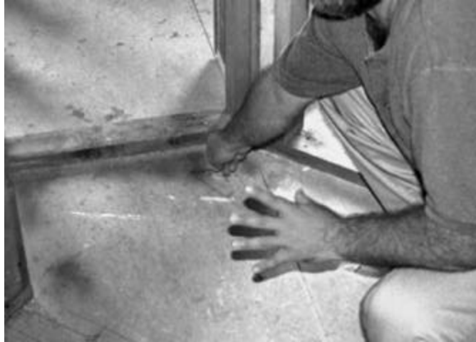
Figure 9 Spray paint marking chase location
