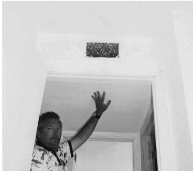
Figure 6 Chase in hallway, note 7'0" ceiling and door clearance
