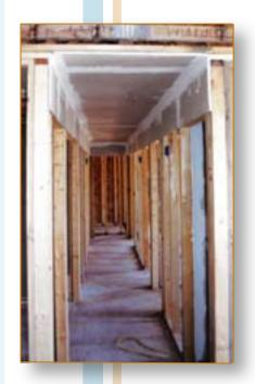
In hallway fur-down chases, the air barrier is installed and sealed on both sides and the top of the chase first.
