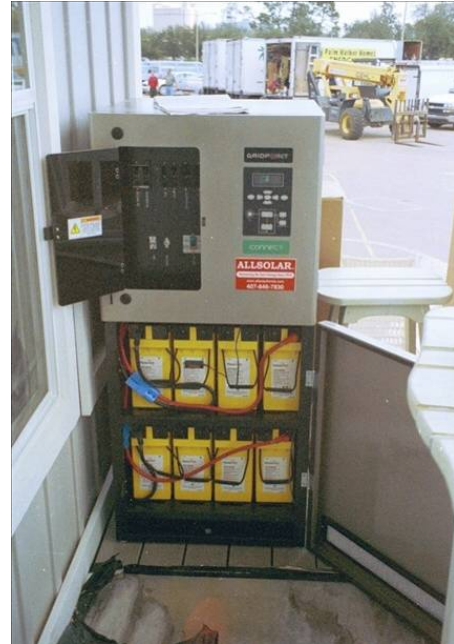
Figure 2-21 GridPoint Invert and battery Back-up Energy Management System
