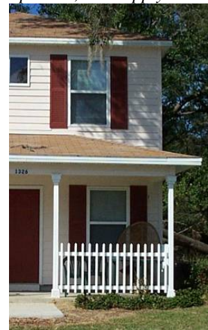
Figure 4-6 Low-E windows are enhanced by two foot overhangs, porches, and site shading.
