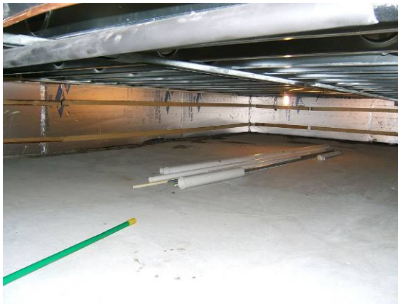
Figure 2- 6 Weather tight and insulated crawlspace
