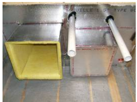
Figure 3-5 Air barrier in top of air handler closet created with duct board by the mechanical contractor at the time that the ducts are installed.
