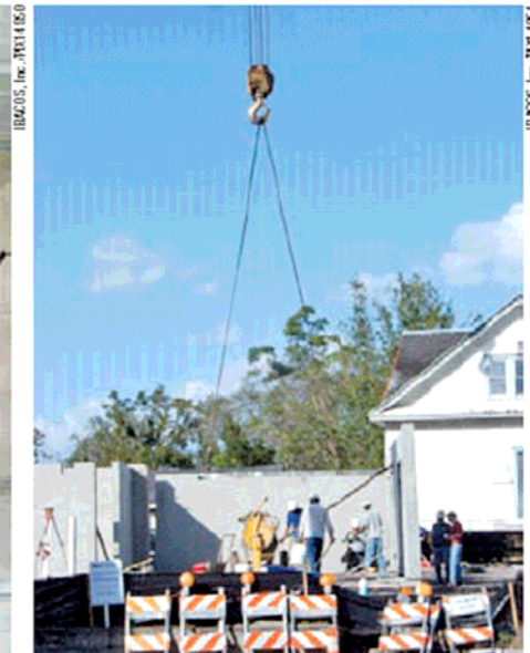
Pre-cast exterior concrete walls allow for faster building enclosure construction and a tighter envelope.
