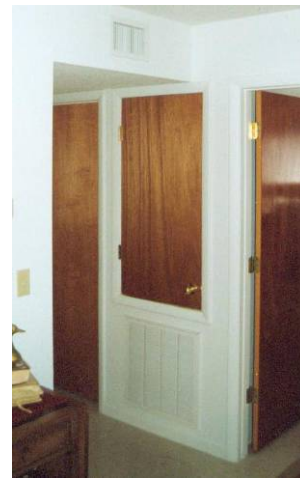
Figure 4-5 A Interior air handler, return plenum, and supply duct chase.
