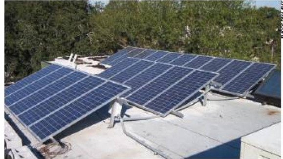
Figure 2-23 2.25kWp Photovoltaic power system on roof top of 2007 TNAH
