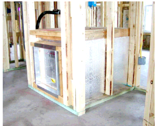
Figure 4-12 Detail of a ducted return air plenum
