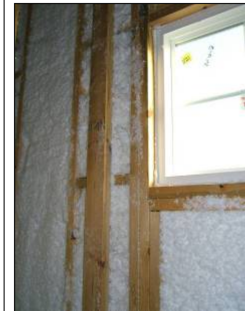
Figure 3-12 Close up of ladder detail at the intersection of an interior wall. "Rungs" provide drywall nailing surface without compromising insulation.
