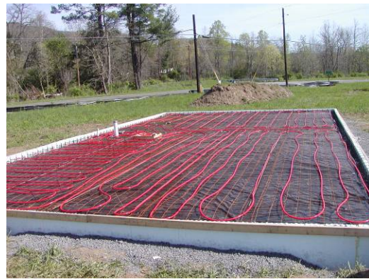
Figure 4-14 Radiant floor system installed prior to slab pour
