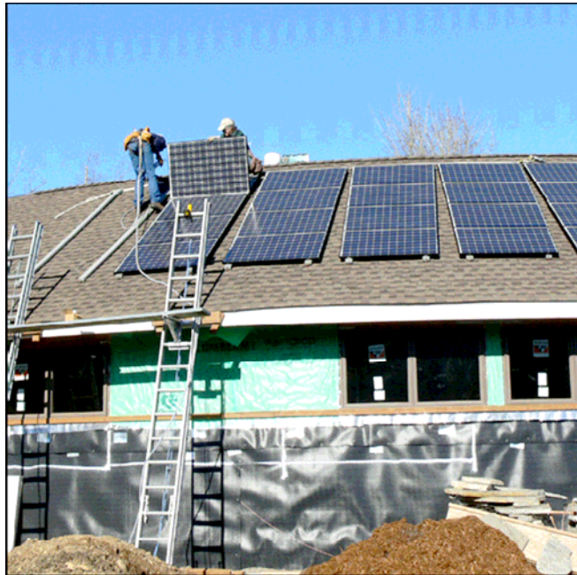
Figure 2-19 PV panel installation, Garst Residence
