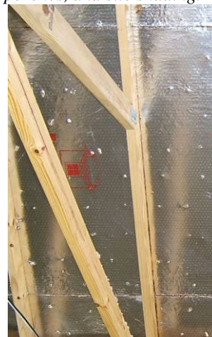
Figure 4-7 Radiant barrier reduces heat transfer from the roof, a major component of the cooling load.
