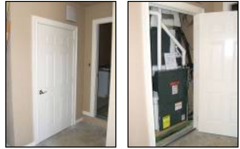
Figure 3-4 Exterior walls around air handler isolate closet from garage, create valuable conditioned square
