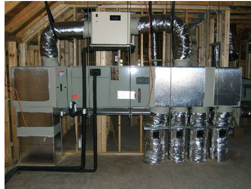
Figure 2-5 HVAC equipment installed
