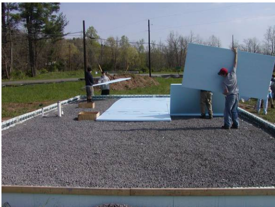
Figure 4-13 Rigid insulation being installed on rock bed within ICF stem wall
