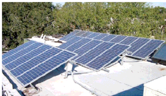
A PV system powers the refrigerator directly, and the excess energy is either used elsewhere in the home or stored.
