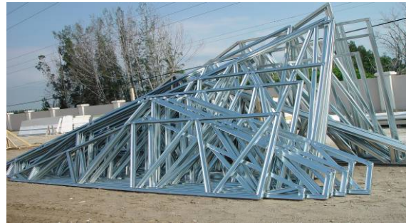
Figure 2-13 Steel trusses produced on site
