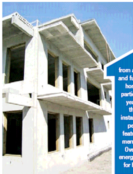
Pre-cast concrete overhangs provide area for vegetation and shade to reduce solar heat gain.
