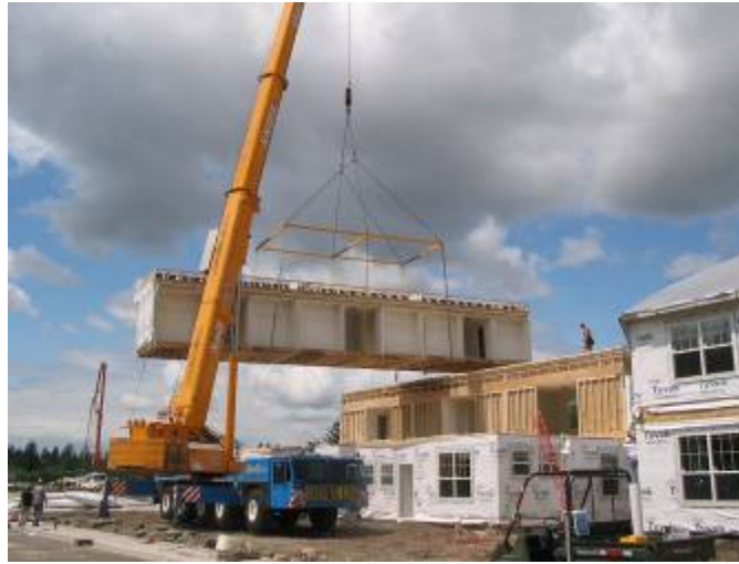
Figure 3-16 Two story Modular housing assembly - Fort Lewis Army Base, Washington
