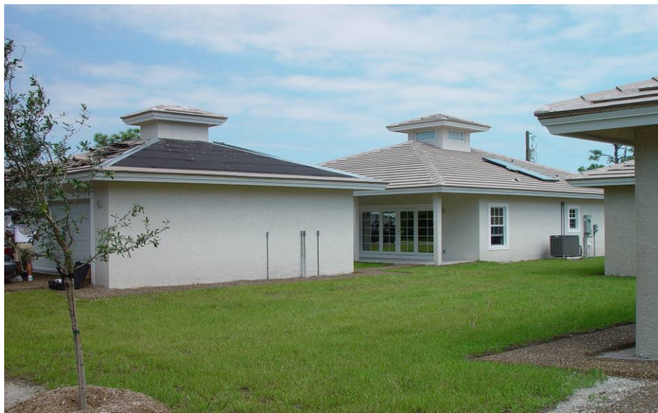
Figure 2-18 Homes with sola hot water and BIPV on detached garage (not installed yet)
