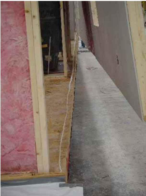
Figure 1-14 Bottom plate airseal inspection – thermal bypass inspection checklist item
