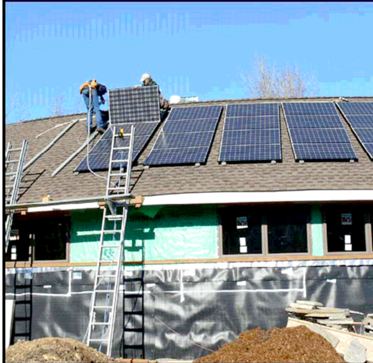
Figure 1 – PV panel installation, Garst residence – Olympia, WA
