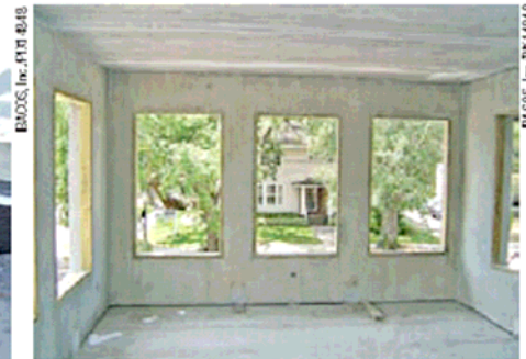
Openings for windows and any other penetrations required careful design and placement in the pre-cast concrete system.
