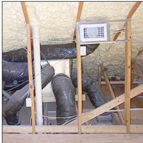
Figure 84 Semi-conditioned space for the ductwork.
