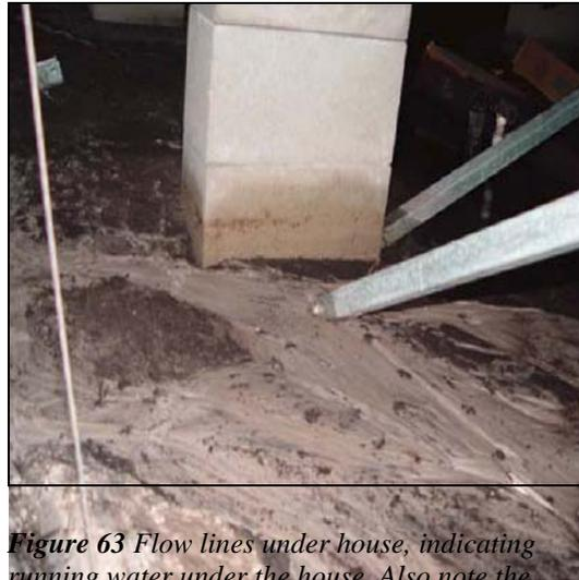
Figure 63 Flow lines under house, indicating running water under the house. Also note the “tide line” on the support column.
