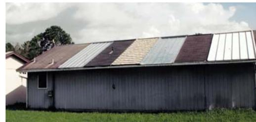
**Figure 104** Flexible Roof Facility in summer 2002 configuration. Cells are numbered from left to right starting with the second cell in from the left.
