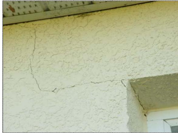
*Figure 90 Window corner crack*
