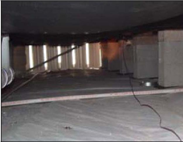
**Figure 65** HUD Code required perforations in skirting may not allow adequate volumes of ventilation, creating higher than usual vapor pressure difference across the floor assembly even though the ground cover and belly board are in good condition.
