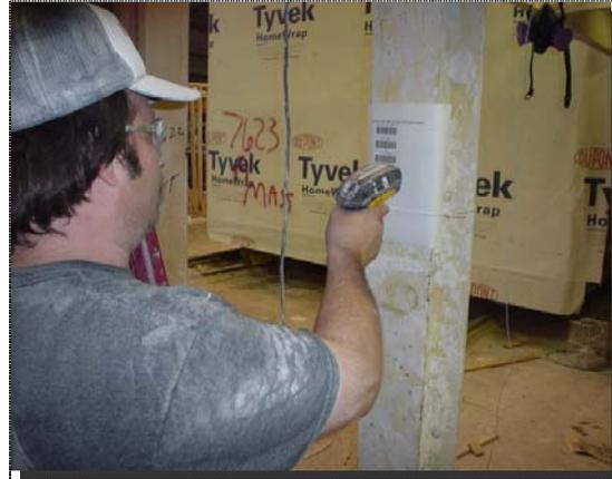
*Figure 51* Scanning drywall activities with new STACS device.
