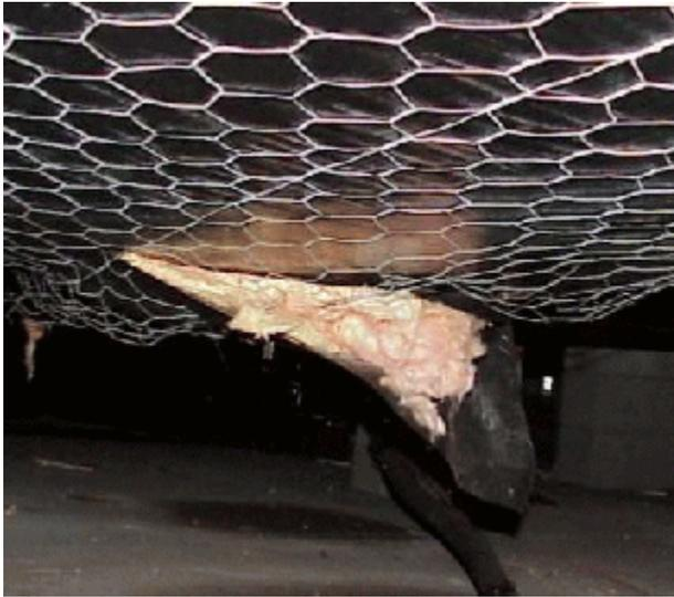
**Figure 49** Another belly tear found during inspection.
