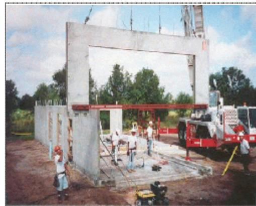
*Figure 54 Setting pre-cast concrete wall panel.*
