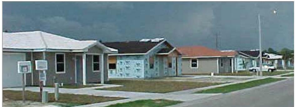
**Figure35** Street scene showing the three closest homes (from left: white "barrel" s-tile (RWB), terra cotta s-tile (RTB) and white metal (RWM)).
