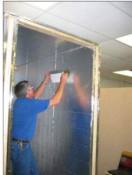
**Figure109** Installing un baffled return air flow through wall grille
