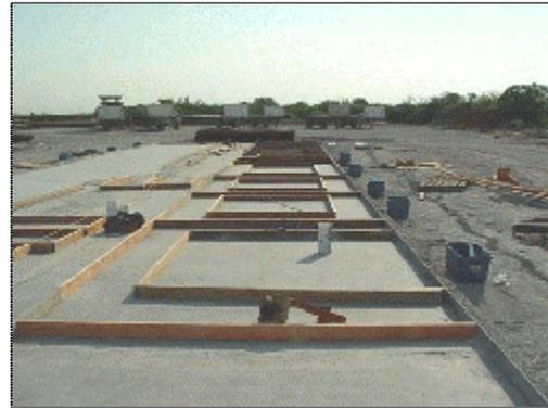
*Figure 53 Panel forms on forming bed.*
