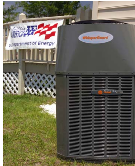
Figure 13 Prototype condenser fan and exhaust housing.
