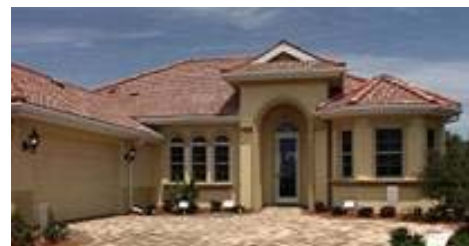
Figure 25 WCI Green home in Venice, FL.
