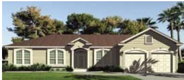
Figure 23 Palm Harbor modular home for the 2005 International Builders Show
