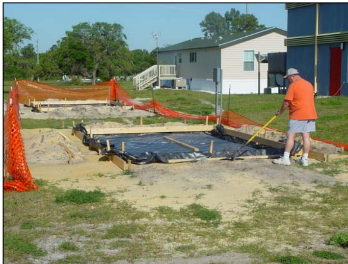
Figure 5. Site location of side-by-side NightCool and basecase test sheds.
