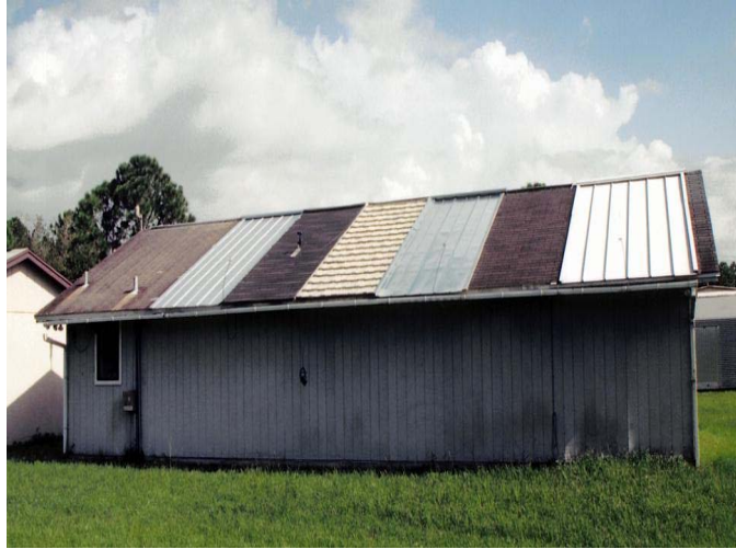
Figure 1. FSEC's Flexible Roof Facility
