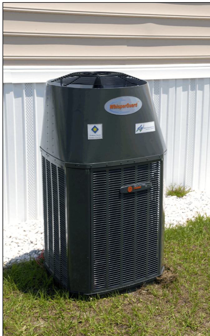
Figure 4. Improved condenser fan with enhanced diffuser.
