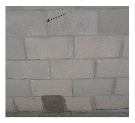
Figure 64 Extended stairstep crack (arrow) on outside wall after grouting cells and installing roof (note that crack extends through vertical grouted cell)
