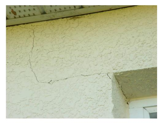
Figure 30 Window corner crack
