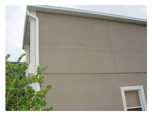
Figure 28 Reparied horizontal crack on 2<sup>nd</sup> floor frame wall
