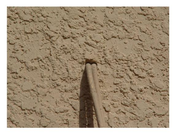
Figure 23 Unsealed penetration for wiring
