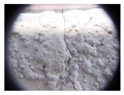
Figure 35 Typical crack between 0.39mm (1/64 inch) and 0.58mm (1/48 inch) wide
