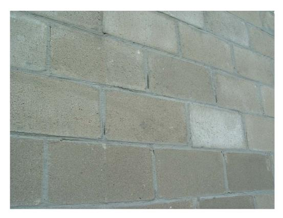
Figure 15 Varying workmanship of mortar joints
