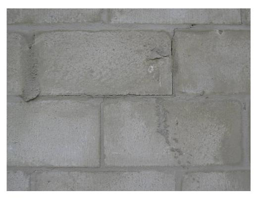
Figure 63 Extended stairstep crack on inside wall after grouting cells and installing roof
