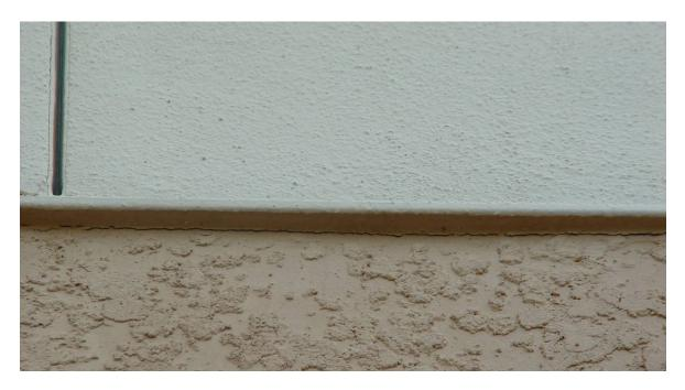
Figure 25 Crack at 1<sup>st</sup>/2<sup>nd</sup> floor expansion joint
