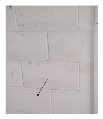
Figure 54 Home #3 showing through-wall stairstep crack (not repaired on inside) and small water leakage out of crack (see arrow)
