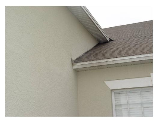
Figure 18 Stucco cracking and damage around flashing
