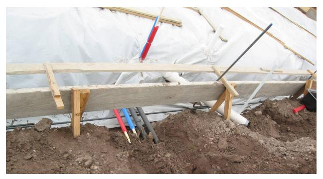
Figure 60 Foundation penetrations for freshwater and drain lines
