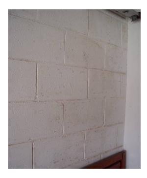
Figure 48 Discoloration in garage from water intrusion during storm
