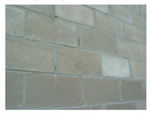
Figure 62 Typical cracks and voids observed in mortar joints in masonry walls
