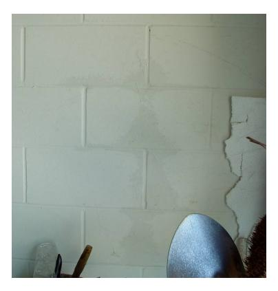
Figure 56 Home #4 showing through-wall stairstep crack and growing dampness
