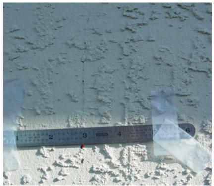
Figure 32 The smallest crack measured - 0.13mm wide
