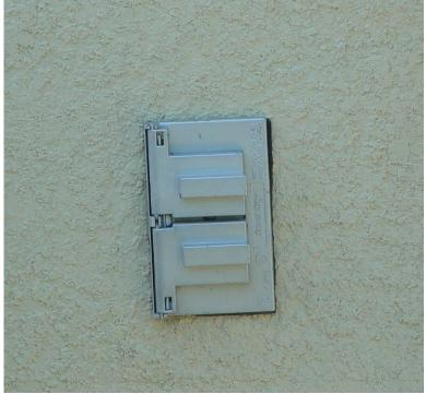
Figure 22 Unsealed penetration for electrical outlet
