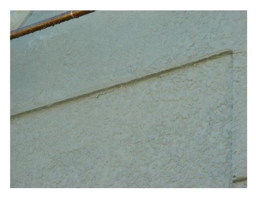
Figure 49 Minor cracking under expansion joint
