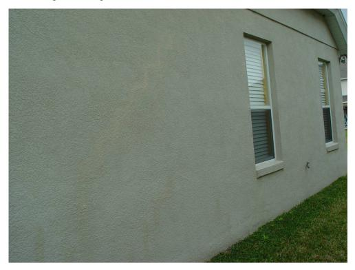
Figure 29 Patch of stairstep crack using elastomeric compound
