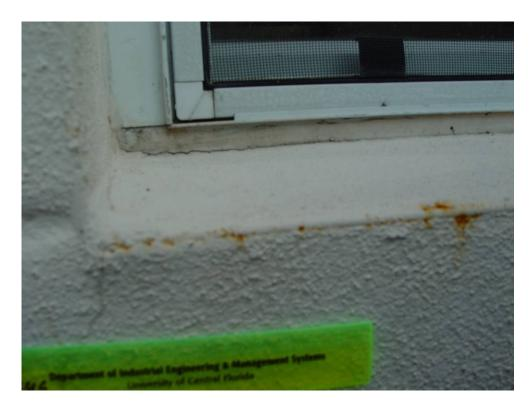
Figure 19 Cracks in window caulking
