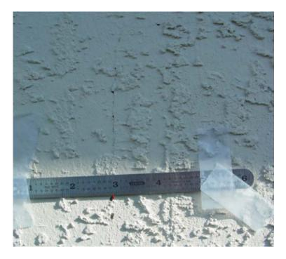
Figure 52 Home #2 with smallest crack measured (0.13mm wide) – testing revealed no intrusion
