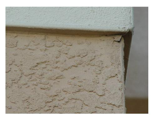
Figure 24 Crack at 1<sup>st</sup>/2<sup>nd</sup> floor expansion joint from poor workmanship
