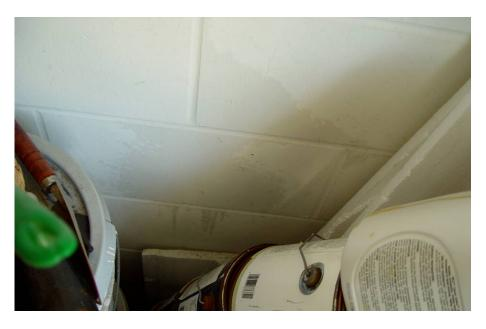
Figure 57 Home #4 growing dampness and drips forming near floor
