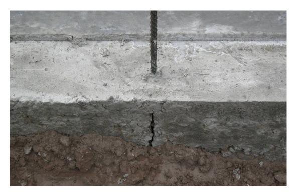
Figure 61 Incomplete concrete pour around vertical steel in foundation
