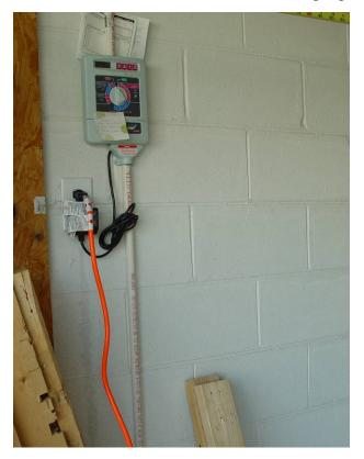
Figure 51 Note leak out of electrical outlet (directly under rain gauge penetration)
