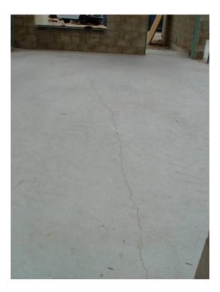
Figure 65 Typical crack in floor slab
