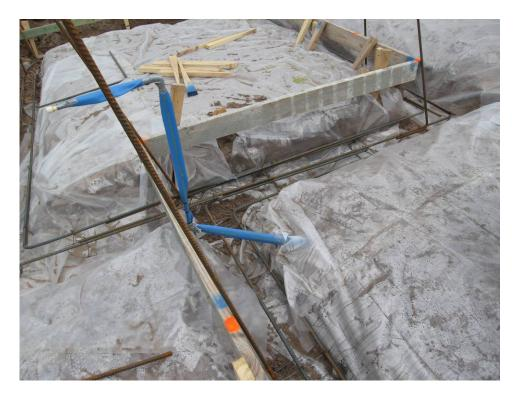
Figure 59 Layout of steel rebar in foundation trench
