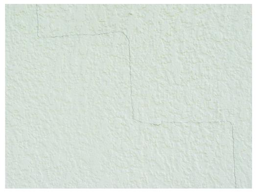
Figure 38 Typical stairstep crack greater than 0.78 mm (1/32 inch) wide
