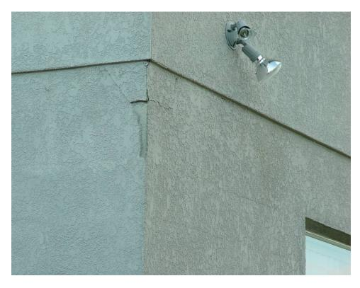
Figure 26 Stucco damage on corner
