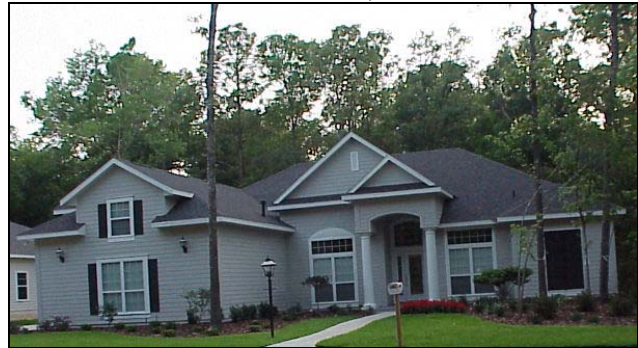
Figure 2. Home built by GW Robinson, Gainesville, FL.
