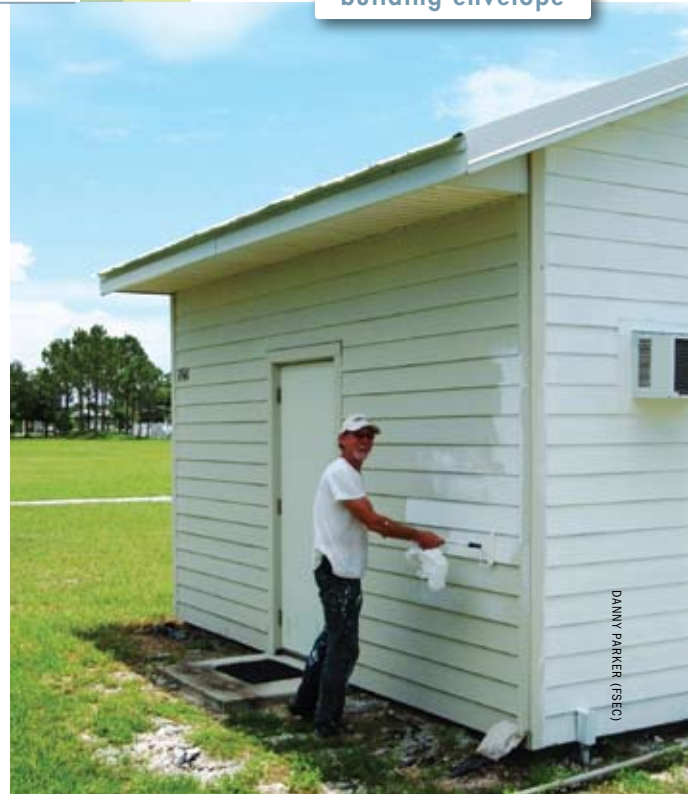
Patrick Gillis adds the first coat of bright white latex paint to the FSEC test building.
