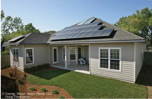
The Galloway Model with 6.75kWp PV and SHW system
