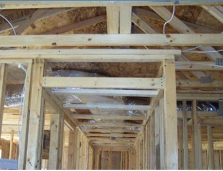
Keeping the airhandler and ducts in conditioned space such as this chase reduces outside air leakage and prevents temperature differences inside and outside the ducts, that can lead to condensation and mold problems.
