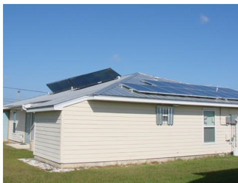
(Left) 40 ft 2 solar hot water and 2.5 kilowatts of PV panels. (Right) Insulated Concrete Form (ICF) walls prior to finishing.
