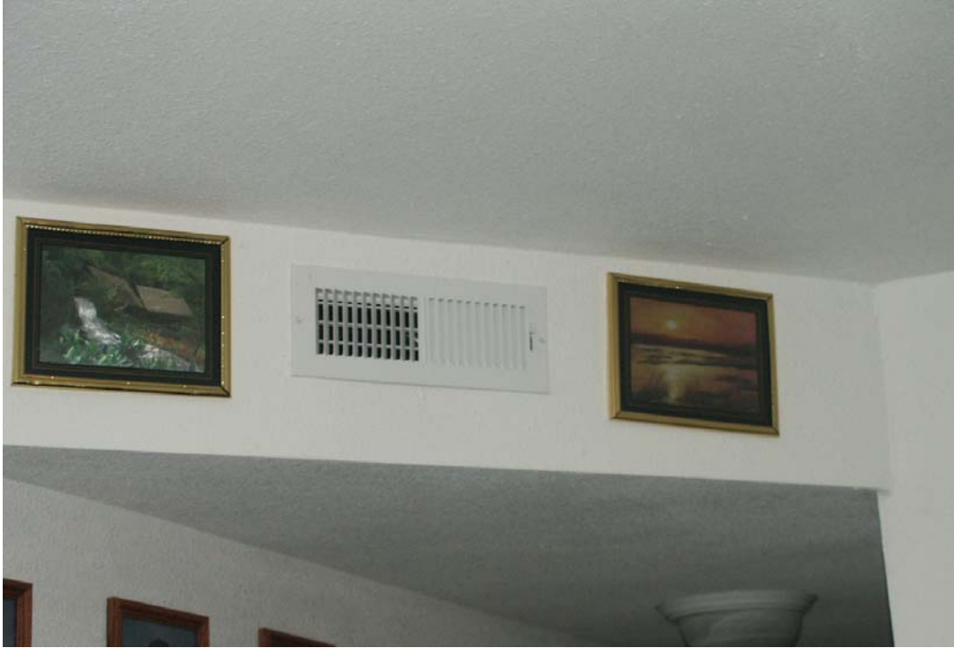
Dropped Ceiling in Hall with Supply Register
