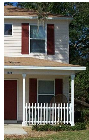
Figure 6 Low-E windows are enhanced by two foot overhangs, porches, and site shading.
