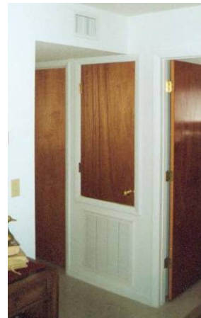
Figure 5 Interior air handler, return plenum, and supply duct chase.
