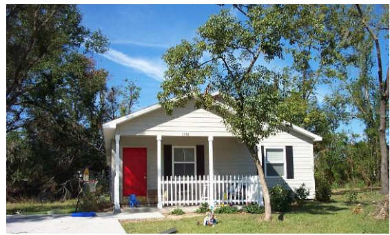
Figure 1. Lakeland Habitat builds one and two story homes of approximately 1100 ft 2 .
