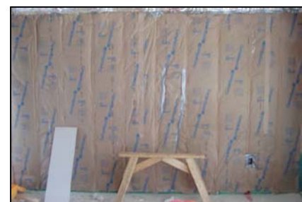
Wall insulation installed with no gaps or compression.
