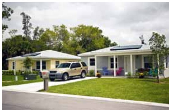
Indian River Habitat’s Grace Woods subdivision features solar hot water heaters to improve energy efficiency.
