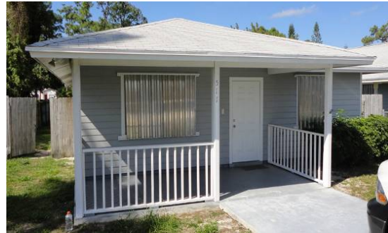
Figure 1. Pre-retrofit with hurricane shutters in place (exterior unchanged during retrofit).
