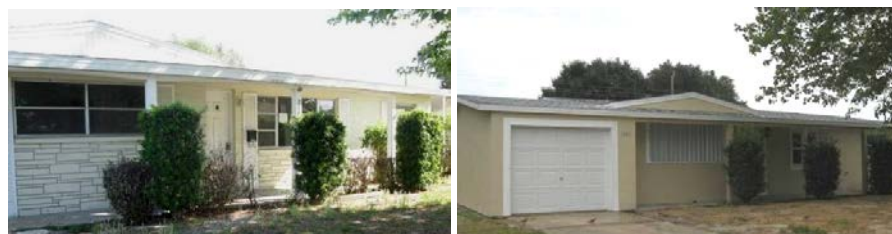
Figures 1-2. Pre-retrofit (left) and post-retrofit (right).
