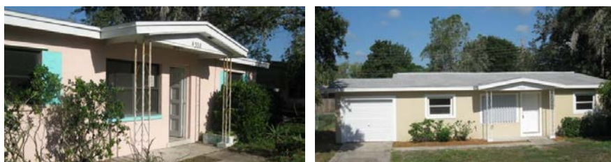
Figures 1-2. Pre-retrofit (left) and post-retrofit (right).
