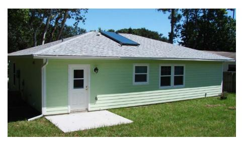
Solar thermal panels, mounted on the south-facing rear roof, provide plenty of hot water at a cost of only \$121 a year to run, compared to \$282 a year for a conventional, 89%-efficient water heater.
