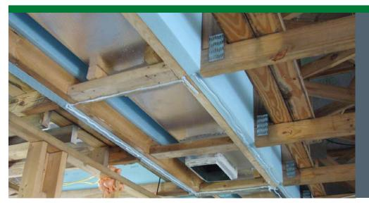
After the rigid foam sides were installed, the rectangular fiberboard duct was lifted into place and supported with 2x4 blocking. Most of the duct registers came directly off the main trunk and boots were installed before raising the duct. The rigid foam chase was further covered with R-11 of unfaced batt for a total chase insulation value of R-31. After the ceiling drywall was installed, R-38 of blown cellulose was blown onto the attic floor around the chase.
