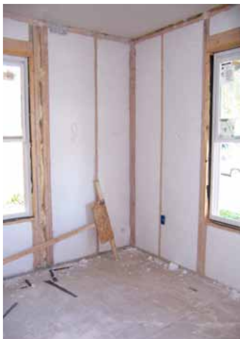
R-13 fiberglass wall insulation blown-in-batt system (BIBS) will not settle or shift over time and fills the wall cavity completely.
