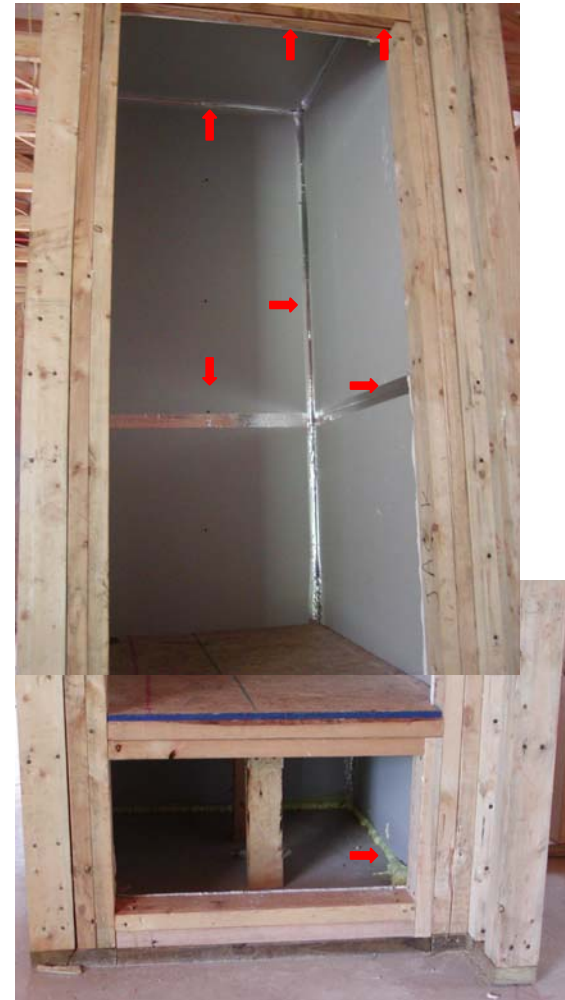
AHU Closet from Inside
