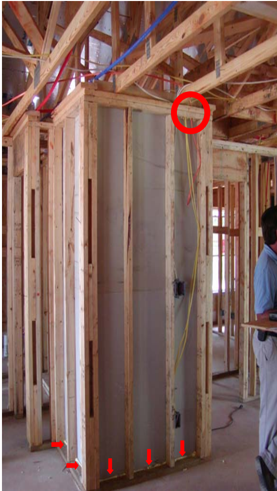
Air Handler Closet from Outside
