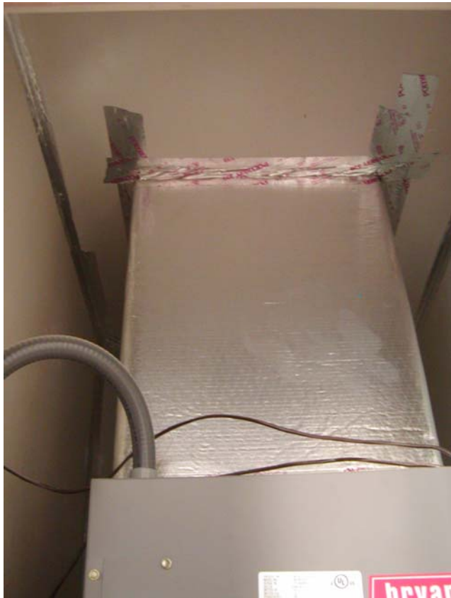
Supply Plenum Sealed to Ceiling
