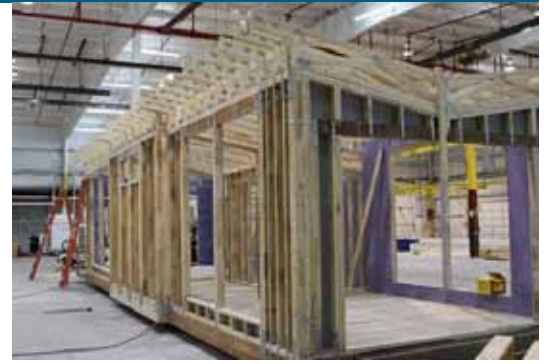
The Osprey Eco Cottage under construction
