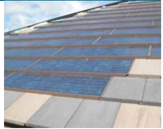
8.0 kW PV System, Flush Mount (160 Integrated 50-Watt Panels)
