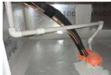
Pre-retrofit: Typical unsealed return plenum (left). Post-retrofit: Return plenum edges and seams are sealed, preventing return air from non-interior spaces, saves energy, and improves indoor air quality (right).
