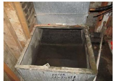
The existing plenum had 4" of standing water from an improperly plumbed condensate line! Replacing and re-plumbing saved energy and improved indoor air quality.
