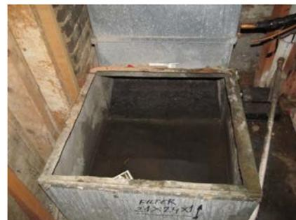
The existing plenum had 4" of standing water from an improperly plumbed condensate line! Replacing and re-plumbing saved energy and improved indoor air quality.
