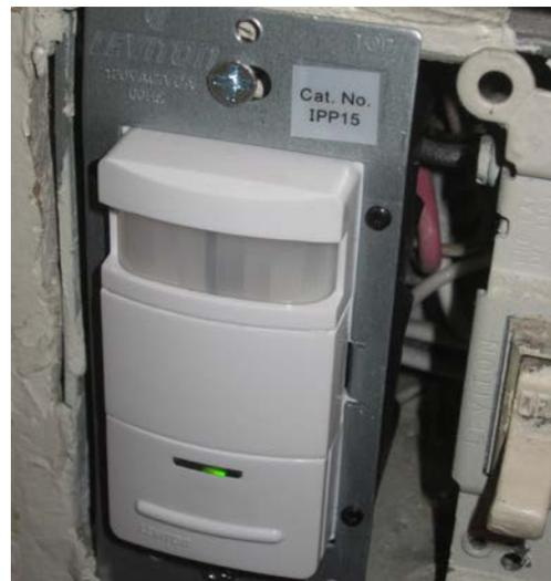
Lighting controls, like this occupancy sensor, helped to automate control and reduce energy consumption.
