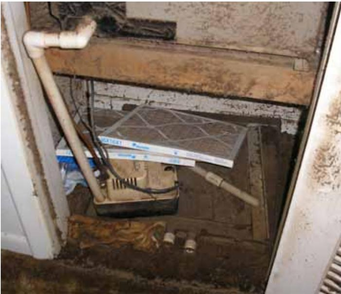
Mold and debris in air handler closet
