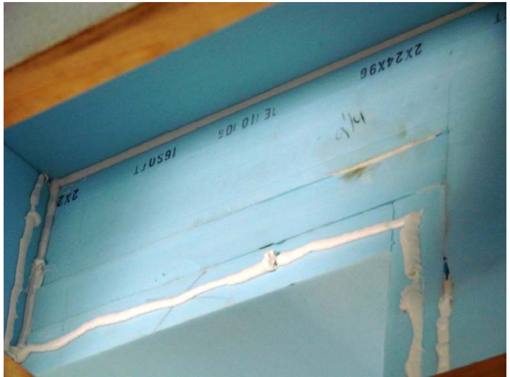
Ready to install the second layer of blueboard. Note the staggered joints and adhesive used to seal seams and attach layers together.
