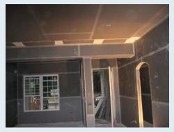
5: Drywall is installed over the chase and the rest of the house, finishing the chase's construction.
