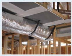
3: Then the supply ductwork is installed under the drywall. The main ducts are hung from the drywall. Rigid ducts are used whenever possible.
