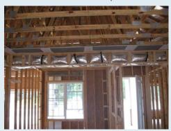
4: The rest of the framing of the chase is now installed.
