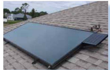
Active solar water heater with (PV) pump
