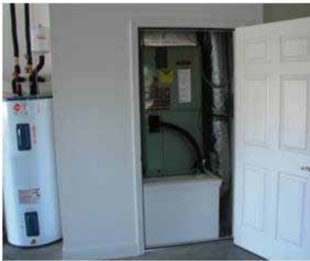
Conditioned handler unit closet access from garage
