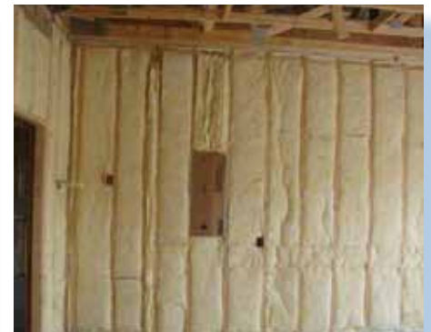
RESNET Grade 1 insulation on frame walls as required by the ENERGY STAR ® Thermal Bypass Checklist
