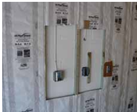
Double battens on block wall allows electric installation without creating penetrations in block
