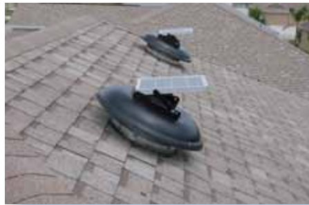
Solar powered attic fans
