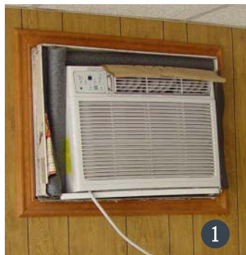
Figures 1-3. Window air conditioning units (1) throughout the building were replaced by 5-ton SEER 15 HSPF 8.7 forced air, central heat pumps (2) and a programmable thermostat for increased energy efficiency. Two externally mounted, natural gas water heaters (3) replaced the three existing electric tank units.
