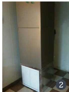
Figures 1-3. Window air conditioning units (1) throughout the building were replaced by 5-ton SEER 15 HSPF 8.7 forced air, central heat pumps (2) and a programmable thermostat for increased energy efficiency. Two externally mounted, natural gas water heaters (3) replaced the three existing electric tank units.
