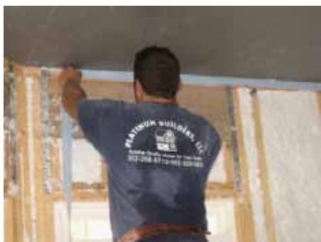
Foam gasket at ceiling/wall joints ensures airtightness
