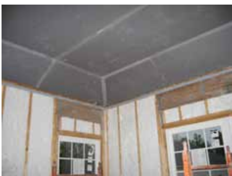
Sealed drywall at ceiling
