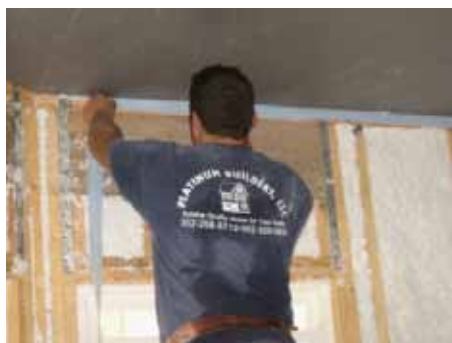
Foam gasket at ceiling/wall joints ensures airtightness
