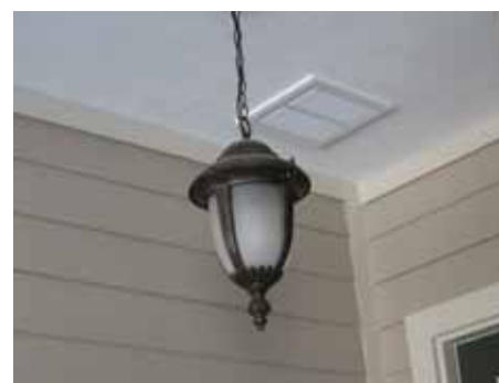
Outside air inlet with filter back grille delivers fresh air to return side of AHU
