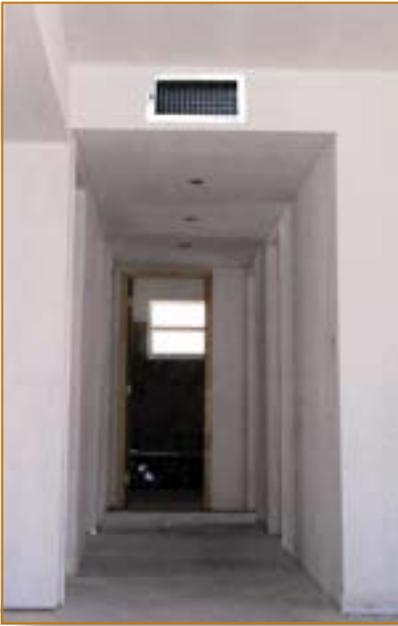
The effect of the lower ceiling height can be offset by increasing the hall width (right).
