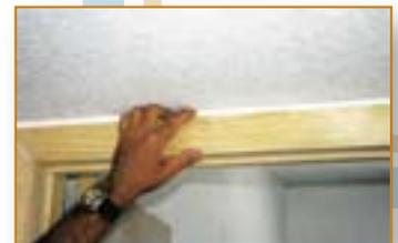
*Code required 7' 0" ceiling height creates tight tolerance for door trim under fur-down chases.*
