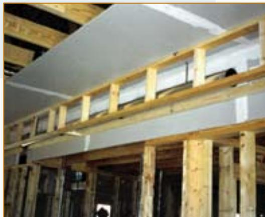
*Fur-down duct chase under construction. Note that chase side extends below framing for the chase bottom.*
