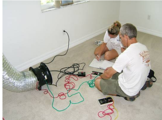
Figure 2-13 Testing Marquis Construction home in Dade City, FL (HERS Index 62)
