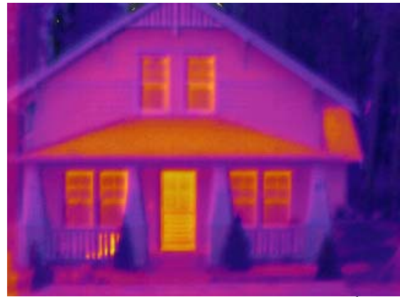
Figure 3-27 Infrared Image of Brotherton 13 th Ave Bungalows
