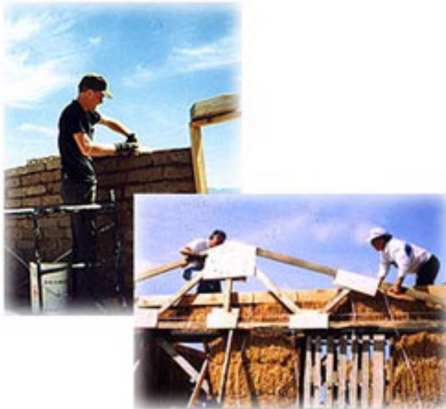
Figure 4-2 Volunteers construct Habitat for Humanity homes
