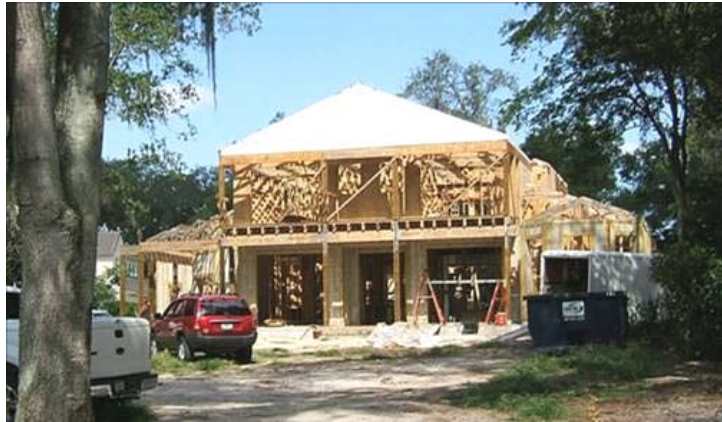
Figure 2-16 Oyler Residence stem wall under construction
