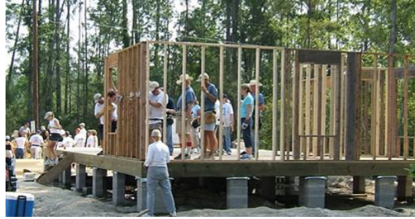
Figure I-17 Raising Walls in a Gulf Coast Habitat Build
