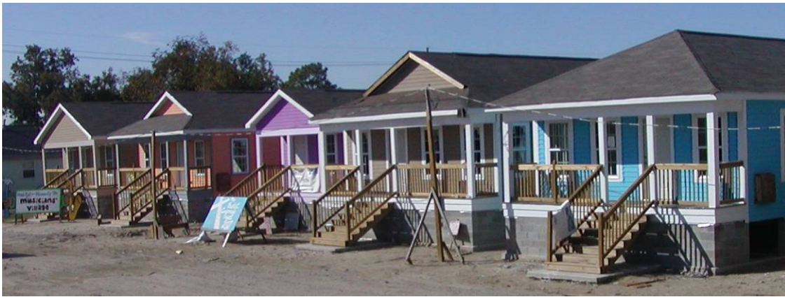
Figure 4-15 New Orleans Habitat Houses
