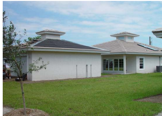
Figure 2-24 Homes with solar hot water and BIPV on detached garage (not installed yet)
