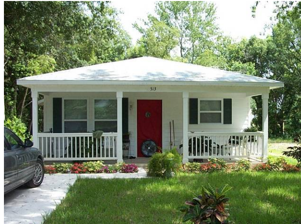
Figure I-16 Lakeland, FL Habitat House under blower-door testing
