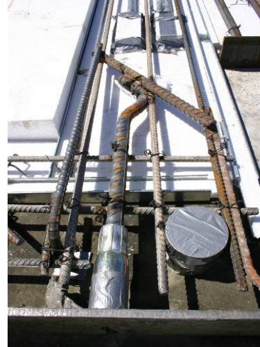
Figure 2-18 Structure & chase details
