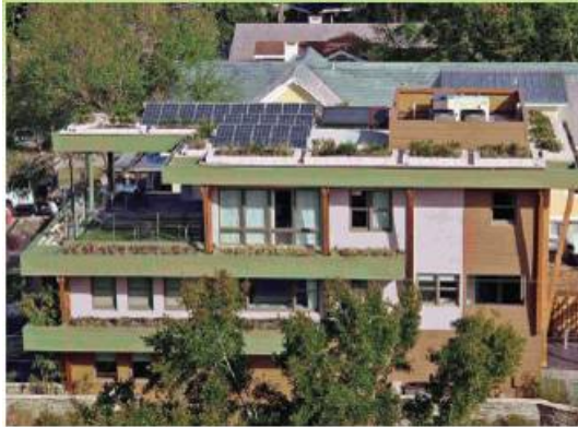
Figure 2-36 2007 TNAH (with the Renewed American Home roof in background)
