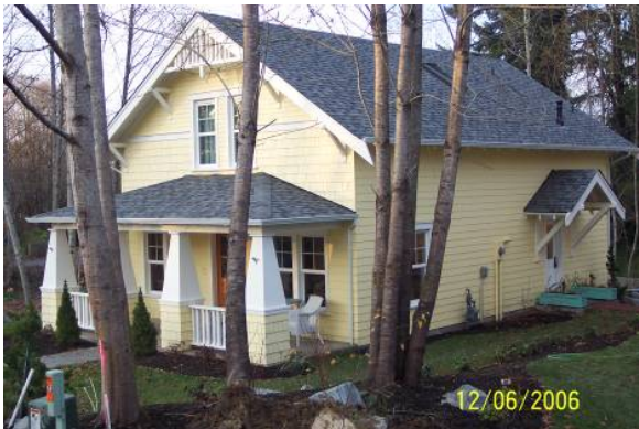
Figure 3-3 Brotherton 13 th Ave Bungalows by Scott Homes, Olympia, WA
