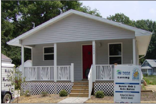
Figure 4-18 JCWP-CBA House built by Lansing (MI) Habitat for Humanity
