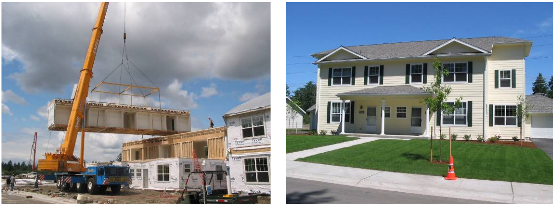
Figure C-11 Two-story Modular Housing Assembly – Ft. Lewis Army Base
