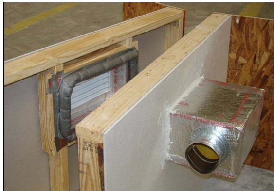
Figure 1-5 Southern Energy Homes Interior Crossover Duct Mockup
