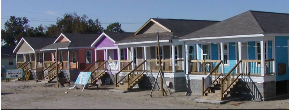
Figure 4-6 New Orleans Habitat Houses
