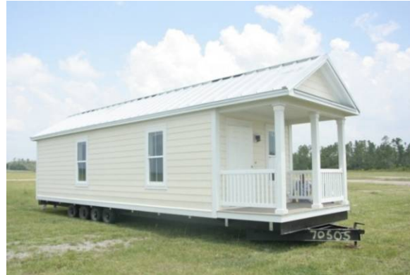
Figure 2-6 FAS Emergency HUD Code Home for Mississippi
