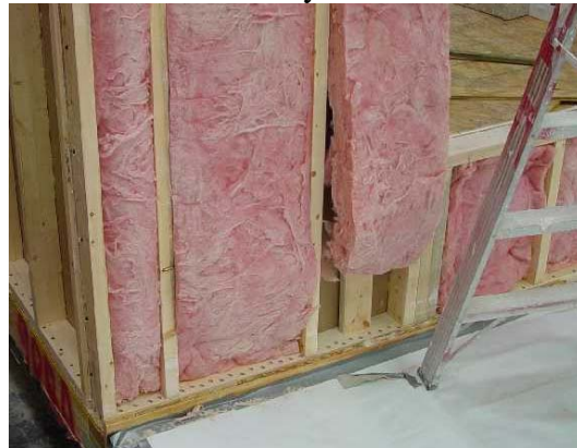
Figure 4-24 Insulation compression inspection – thermal bypass inspection checklist item
