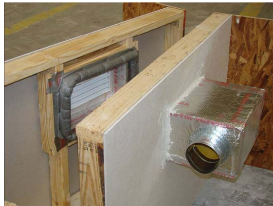
Figure I-6 Southern Energy Homes Interior Crossover Duct Mockup
