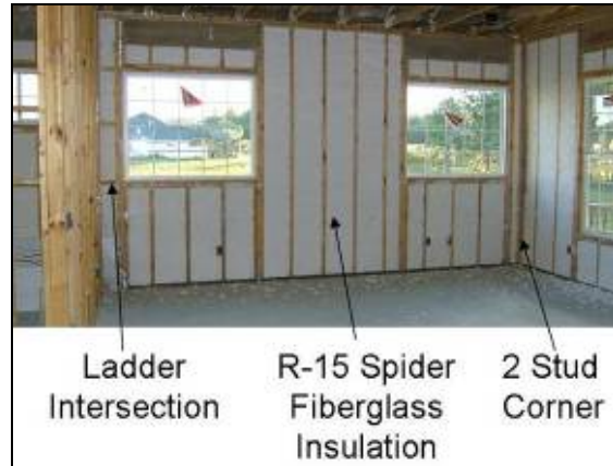
Figure 3-18 Details reduce framing fraction and improve comfort.
