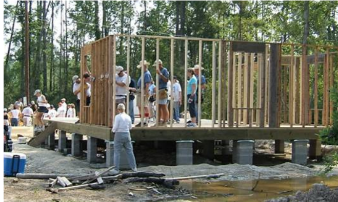
Figure 4-12 Raising Walls in a Gulf Coast Habitat Build
