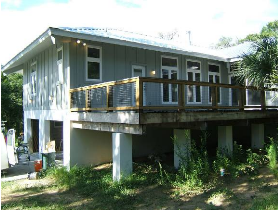
Figure 2-12 Back view of Marquis Construction home in Dade City, FL
