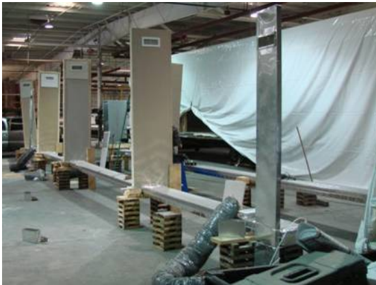
Figure 1-2 Floor duct system with high side discharge outlets under construction being tested with duct tester
