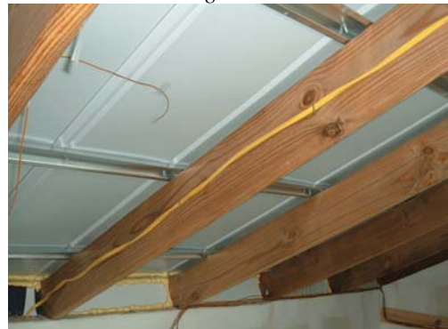
Figure 1-19 Exposed Metal Roof in NightCool Attic
