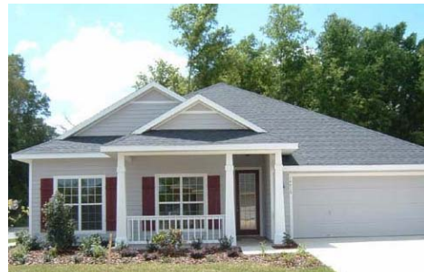
Figure I-13 Turnberry Lake Home
