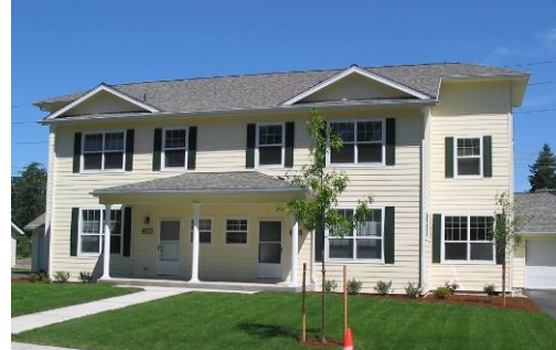
Figure I-14 Two Story Modular Housing – Ft. Lewis Army Base, WA
