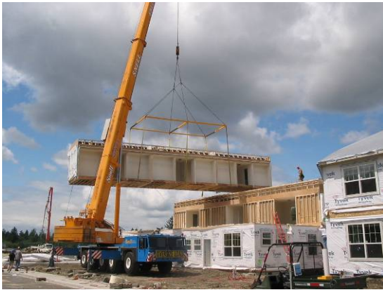
Figure 3-24 Two Story Modular Housing Assembly, Ft. Lewis Army Base, WA
