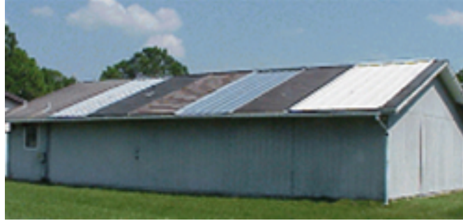
Figure 1-14 The FSEC Flexible Roof Facility (FRF)
