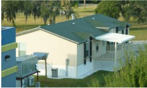
Figure 1-8 The FSEC Manufactured Housing Lab
