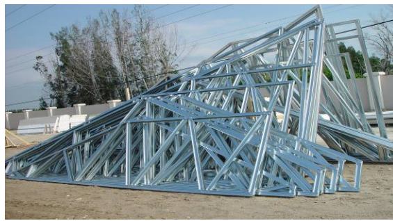
Figure 2-23 Steel trusses produced on site
