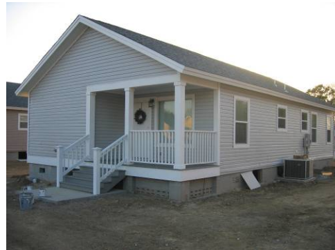
Figure 4-13 Palm Harbor Homes built in Alabama for Oprah Winfrey-HFH partnership
