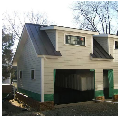
Figure 2-26 Terry Hill House, a high performance residence near Washington D.C.
