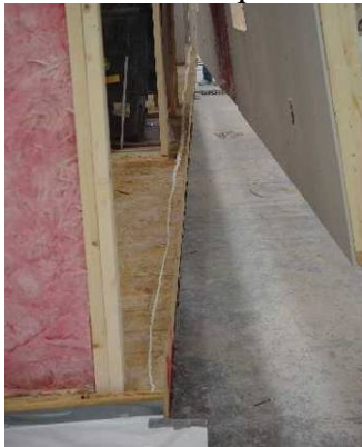
Figure 4-23 Bottom plate air seal inspection –thermal bypass inspection checklist item
