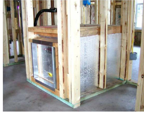
Figure 4-19 Detail of a ducted return air plenum
