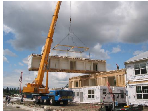
Figure 3-4 Two Story Modular Housing Assembly, Ft. Lewis Army Base, WA
