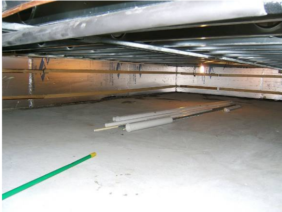
Figure 2-10 Weather tight and insulated crawlspace
