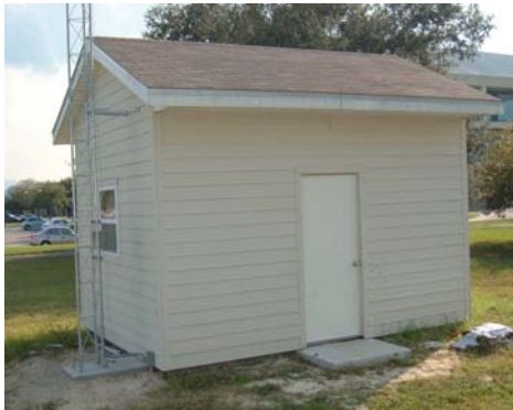
Figure 1-16 Conventional Shed with Dark Shingle Roof
