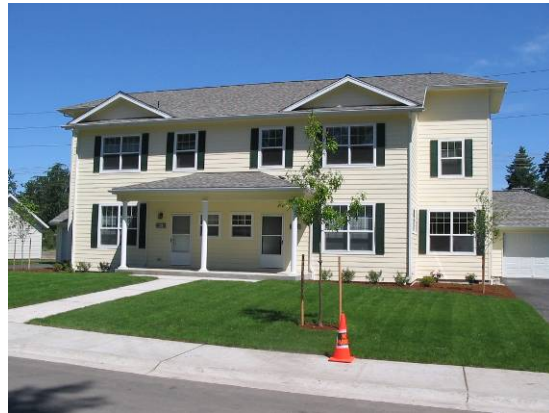
Figure 3-25 Two Story Modular Housing – Ft. Lewis Army Base, WA
