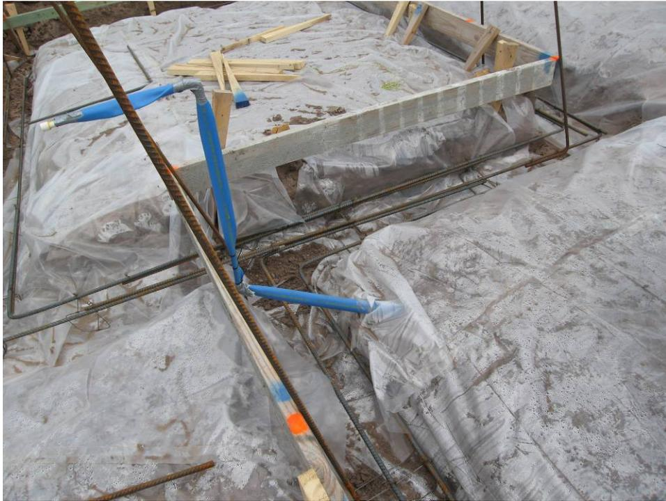
Figure 59 Layout of steel rebar in foundation trench
